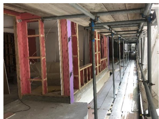
Level 2 Framing around corner steel posts
