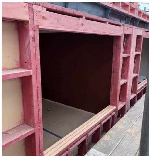
Framing around window openings level 3
