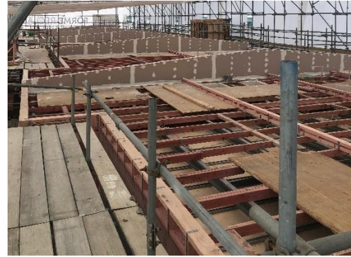
Roof level IT walls
