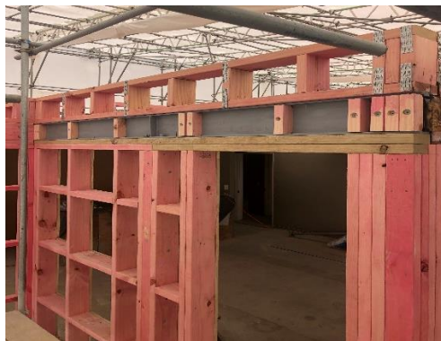
Level 3 Framing and packing out
