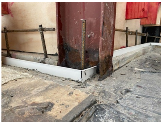
Example of corrosion to steel frames
