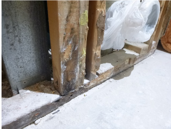
Example of decay and mould in walls to bathrooms
