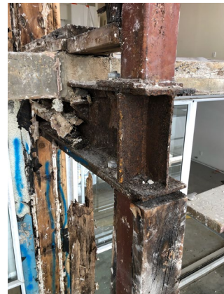
Example of decay and corrosion to external walls
