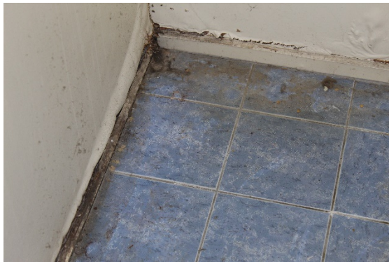
Example of decay and wall damage to walls to bathrooms
