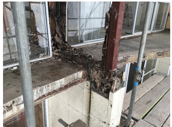
Example of decay to external walls
