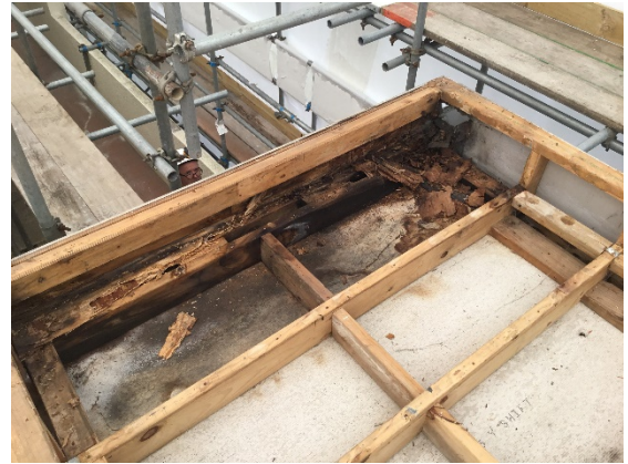
Example of decay to external walls
