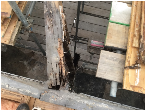
Example of decay to external walls
