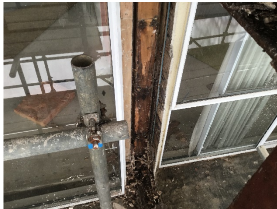
Example of decay and corrosion to external walls
