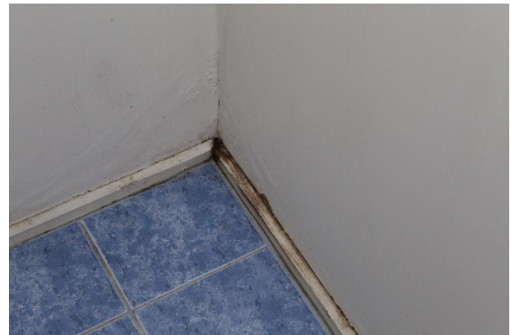
Example of decay and wall damage to walls to bathrooms
