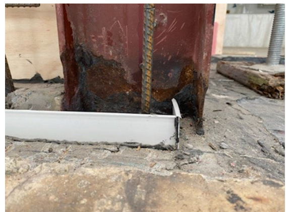
Example of corrosion to steel frames
