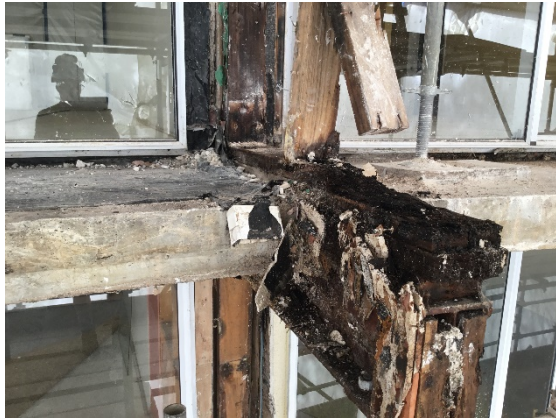
Example of decay to external walls
