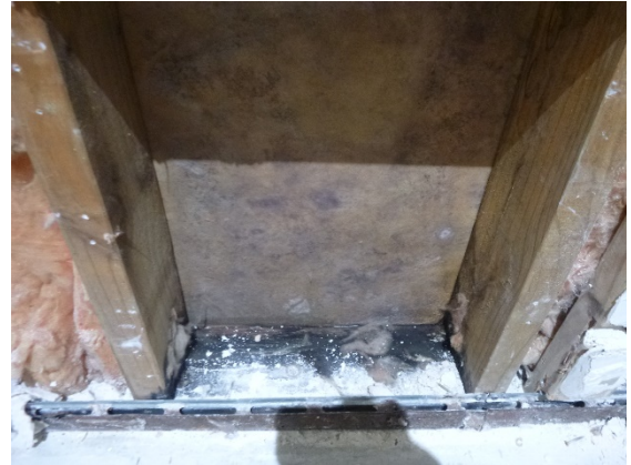
Example of decay and mould in walls to bathrooms
