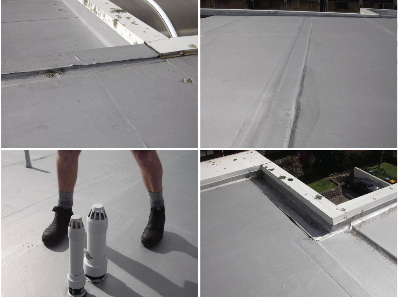
Figure 1 - Grey roof membrane
