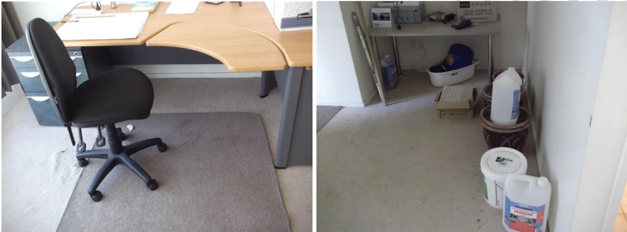
Figure 7 - Flooring to Managers Office
