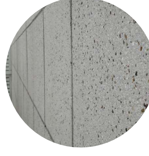
Shotblasted pavers pavers
