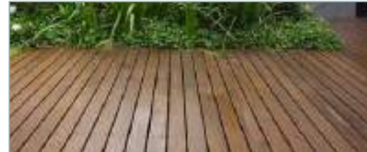
Slatted timber deck (SD)
